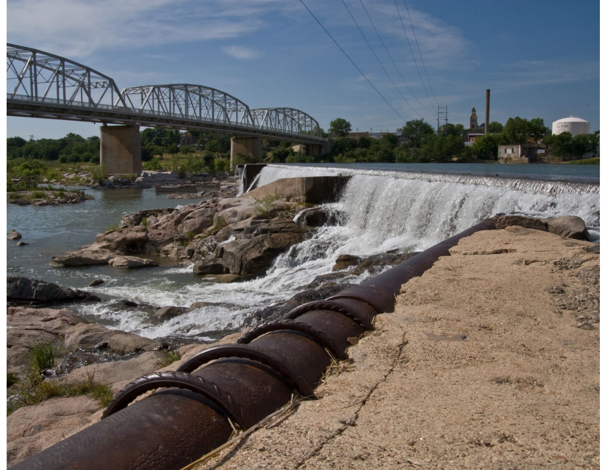
Dam on the Llano River under Hwy 16 in Llano, Texas.
